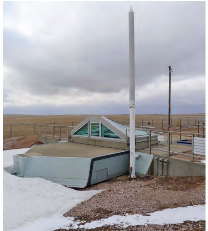
Topside view of D-9 LF showing the greenhouse built to give visitors a view of the missile in the silo
